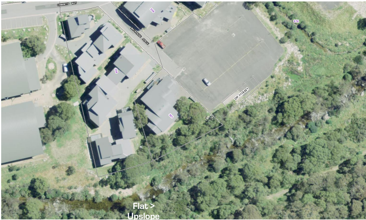
Figure 13: Aerial map showing the vegetation that would have the most influence in the event of a bushfire and its slope
